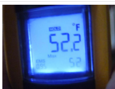
10.0.A Item 2 (Picture) Supply Air Temp
