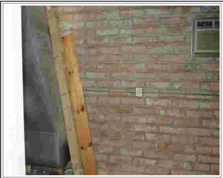
Storage/cooler area on east side
